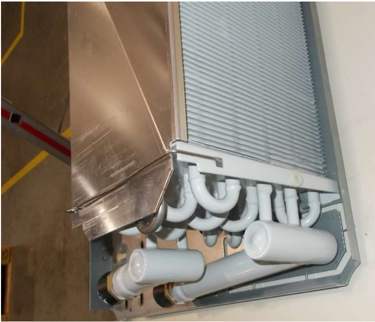
2.5 Mount the defrost water sheet
