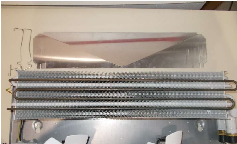
2.3 Put the heating rod in the prepared recess
