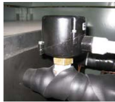
Figure 2 Flow Switch
